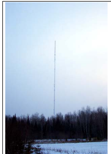
Public Safety Communications Tower (off Church Corner Road)
